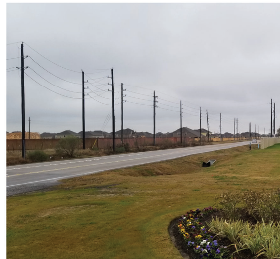
AT ADRIATIC DR FACING EAST, LOOKING SOUTH ON PORTER RD (@ APPROXIMATELY 15-FT SETBACK)
