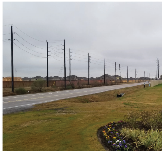
AT ADRIATIC DR FACING EAST, LOOKING SOUTH ON PORTER RD (@ APPROXIMATELY 25-FT SETBACK)
