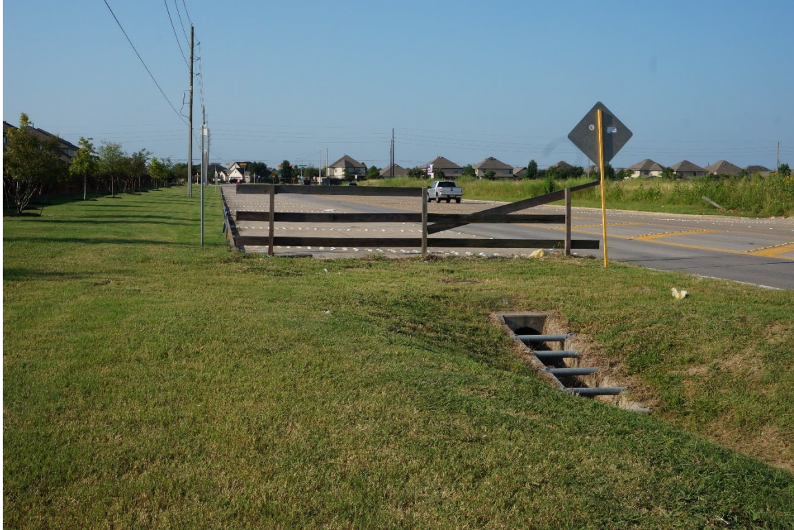
Photograph 3: Transition from four-lane to two-lane road (looking south)
