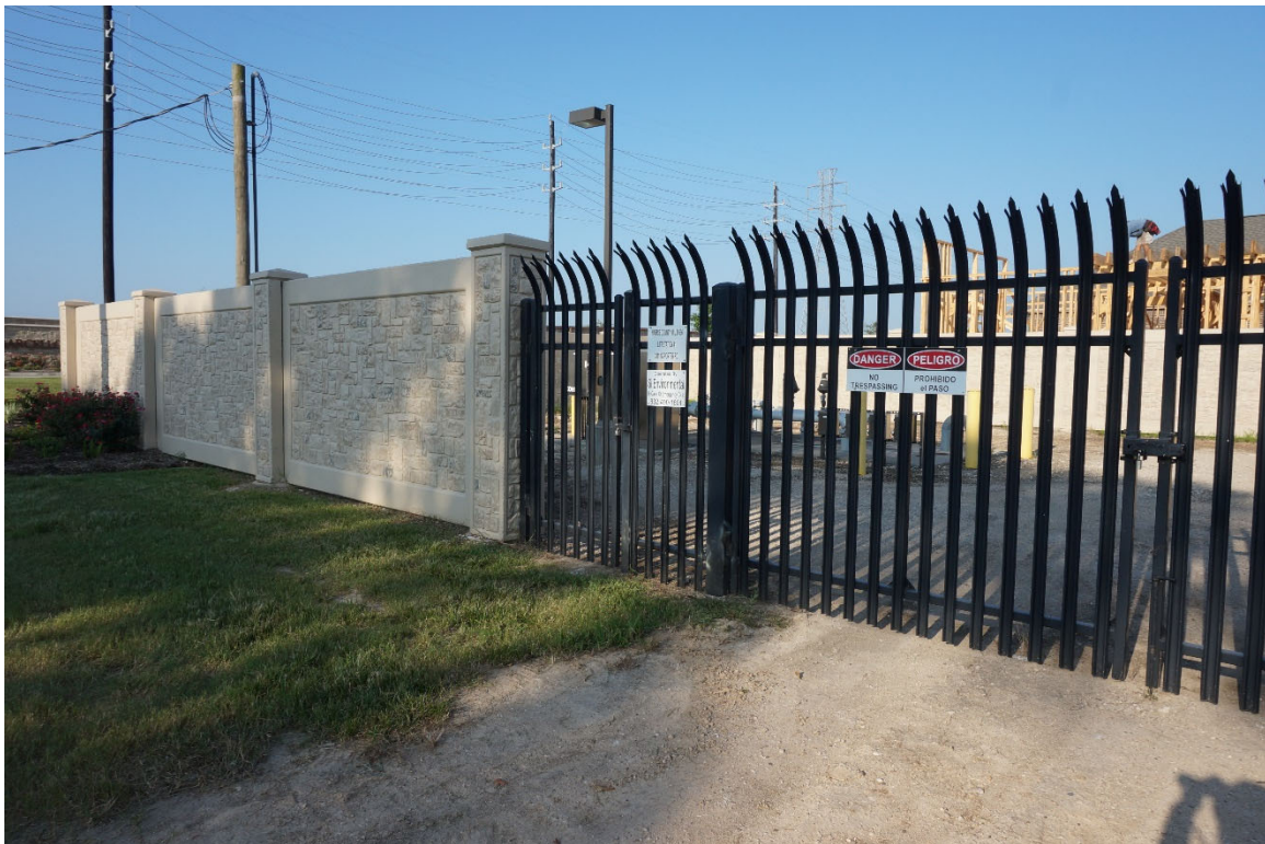
Photograph 12: Harris County MUD No. 536 Lift Station #1 (3311½ Porter Road)
