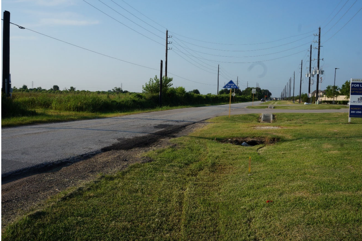
Photograph 7: Creosote telephone poles with pole mounted transformers
