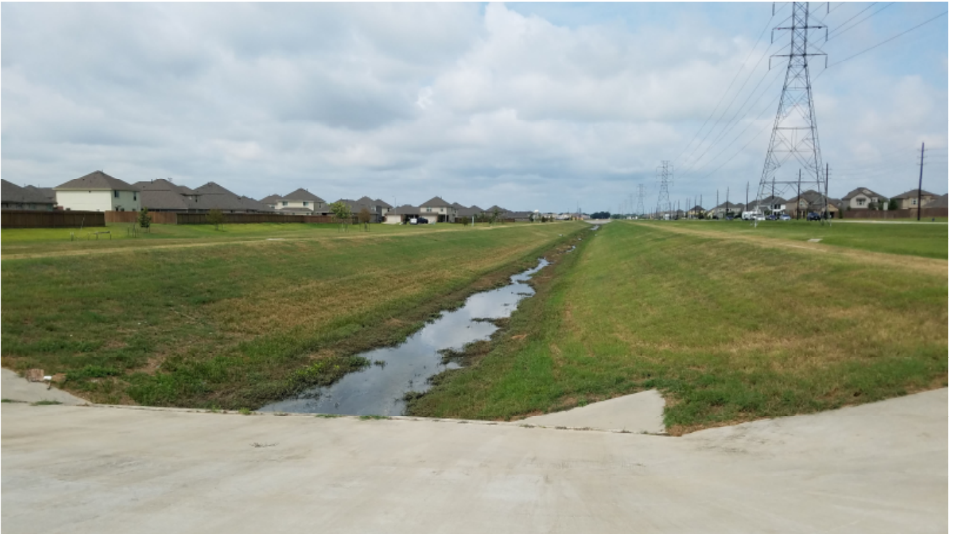
Drainage channel - viewing west on west side of Porter Road
