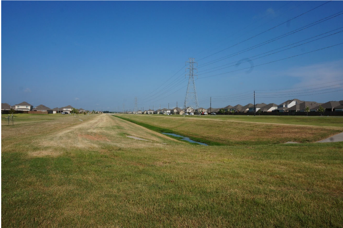
Photograph 8: High voltage power lines running along Harris County drainage canal between northern and southern segments.
