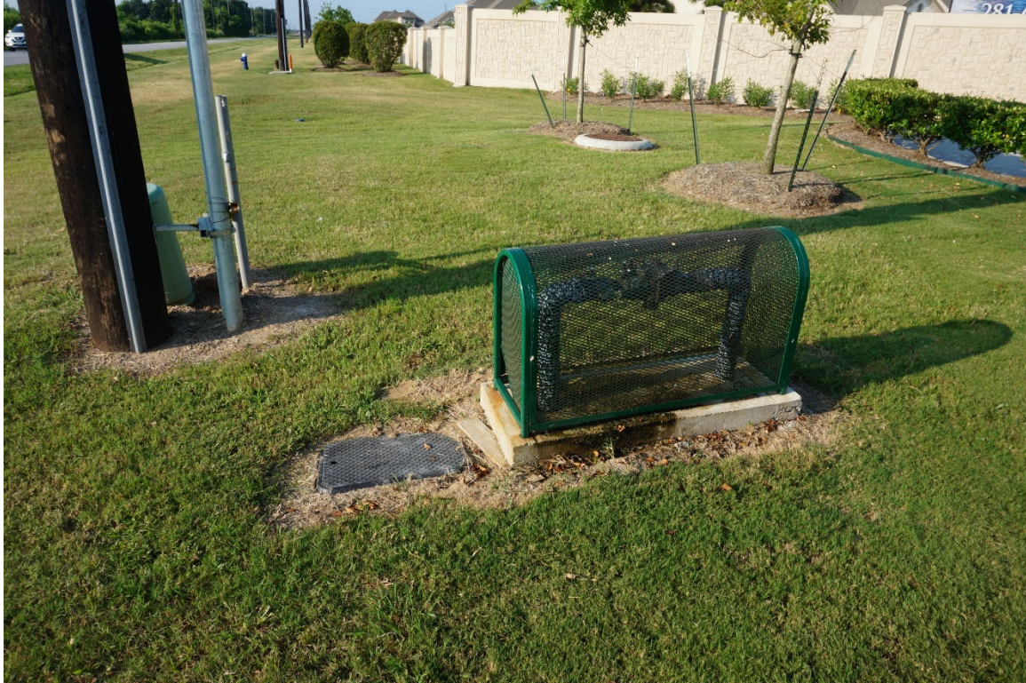
Photograph 19: Above-ground gas line cage, utilities, and residential stone fencing with landscaping
