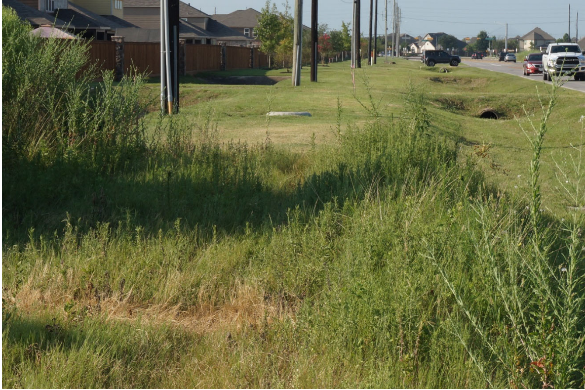
Photograph 21: Small stormwater diversion (on left); short distance has two drainage ditches (near Civitan and Treviso Gardens Road) adjacent to the water treatment plant
