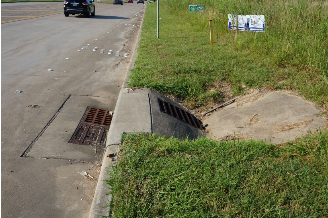
Photograph 4: Grated drainage inlets along curbed roadway
