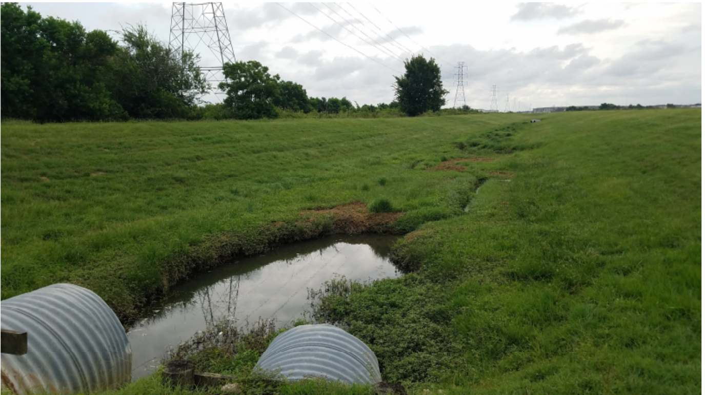
Drainage channel - viewing east on east side of Porter Road (SP3)
