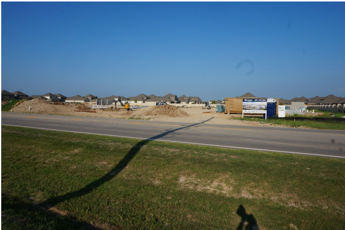
Photograph 22: Commercial property under construction (3315 Porter Road)
