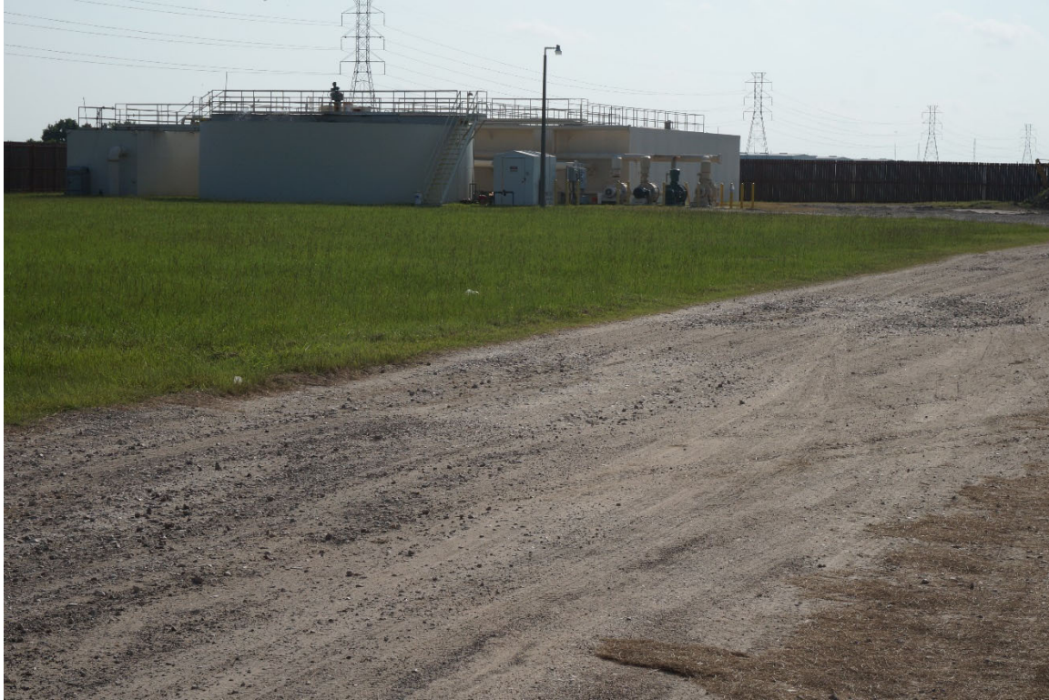
Photograph 13: Harris County MUD No. 432 Wastewater Treatment Plant (3414½ Porter Road)
